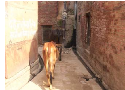
Open House-drains reducing road width
