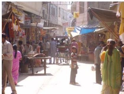
Encroachment on road by the overhangs of the adjoining shops
