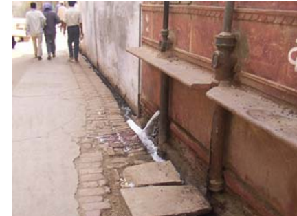
Toilet wastes discharged directly on the roadside drain
