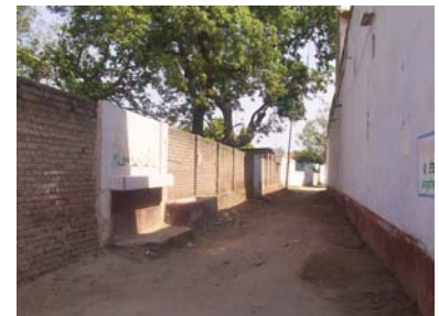
Drinking water facility without drainage
