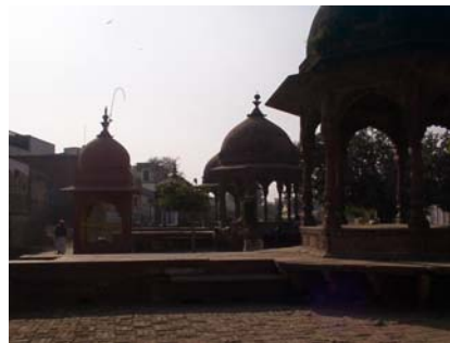
Absence of signage resulting in less attraction
