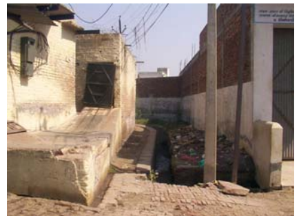
Dumping in Drains running between narrow stretches
