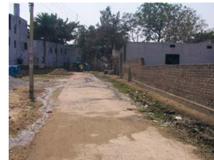
Kutcha Drains on road ID 15
