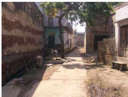
Irregular paving on roads
