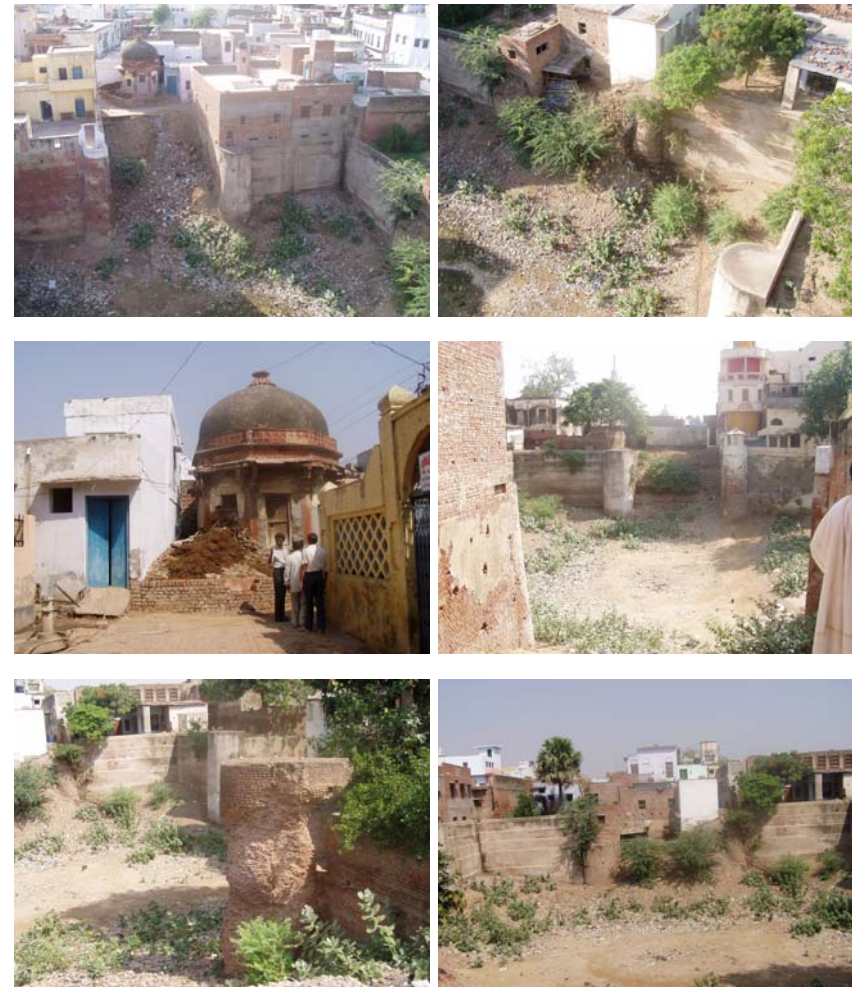
Existing condition of Bramha Kund Potential for Revitalisation
