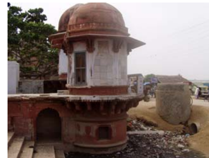
Stagnant drain with Garbage
