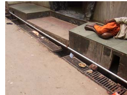
Drains with Metal Gratings
