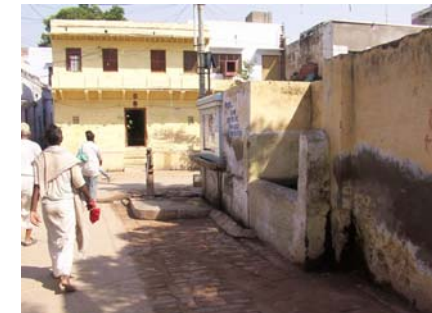
Public Water taps and Hand pump encroaching on the road ID 6
