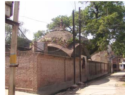
Visual obstructions by Utility lines and High walls
