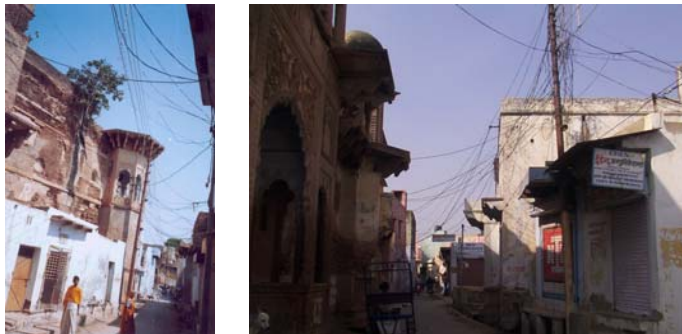
Indiscriminate Overhead Electrical Cable Lines Creating Hazards and Visual Nuisance
