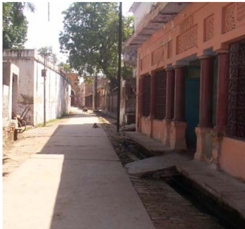
Overhangs over the open drains
